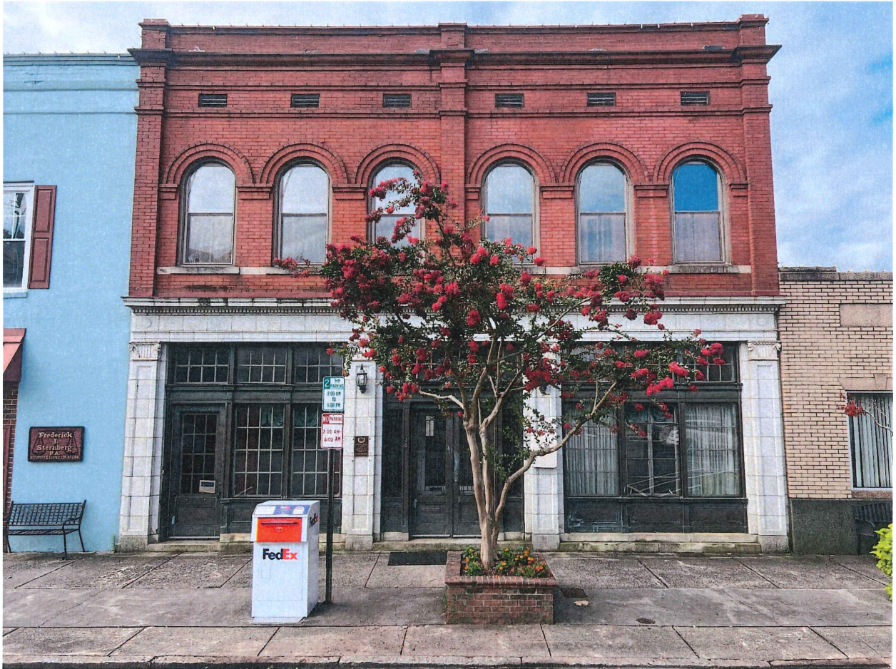
36 Court Square SW - Current photograph
