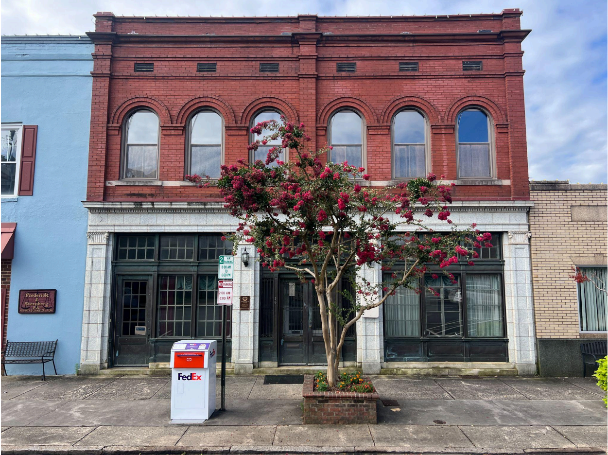
36 Court Square SW - Current photograph
